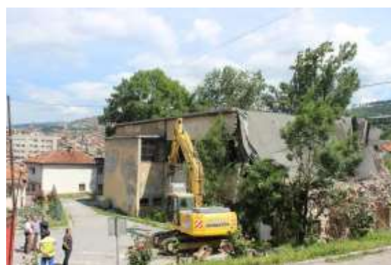
Figure 8: Removal of the old bottom station building (2016)
