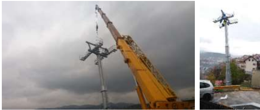
Figures 16&17: Mounting of the tower S3
