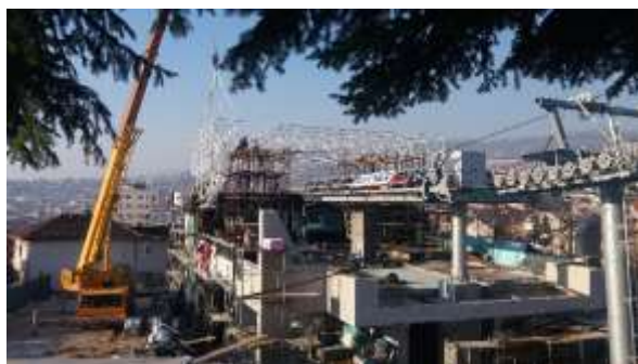
Figure 22: Assembly of the space truss at the bottom station
