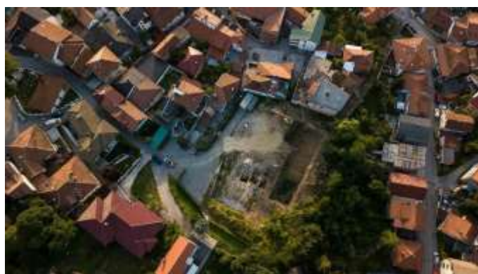
Figure 15: Preparation of the construction pit for the bottom station foundations, viewed from the air
