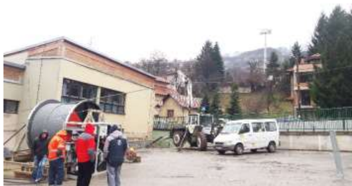
Figure 18: The reel with the main rope during the rope installation process
