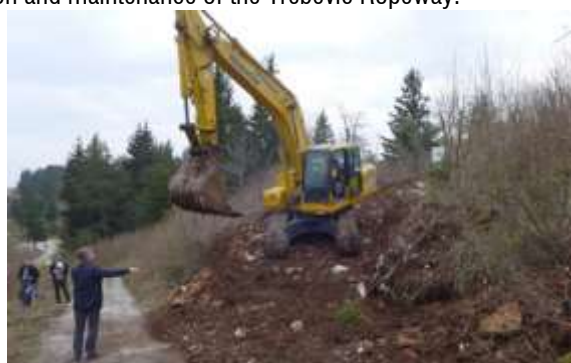
Figure 7: Cleaning of the site at the top station (2015)
