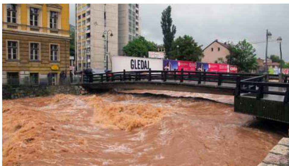
Figure 5 – Floodings in Sarajevo, Bosnia - Herzegovina, source (Al Jazeera Balkans)
