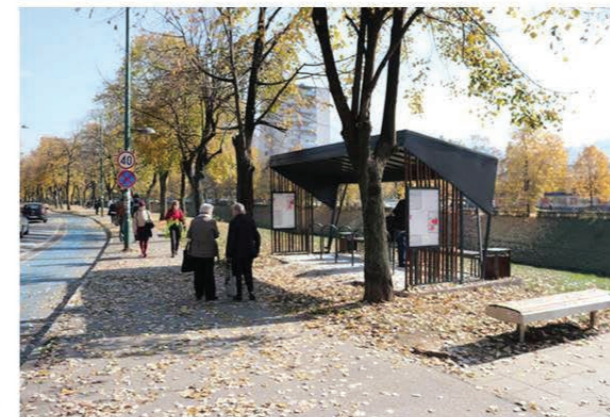
New project construction of covered bicycle parking at nine locations
